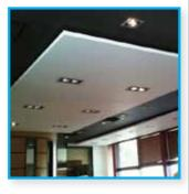
The system is designed around a simplified core set of primitive shapes and modules. When combined, these core shapes provide an extremely innovative and flexible method of construction capable of delivering ceiling rafts in an unlimited number of designs.
