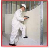
is installed when superior fire protection is required.
