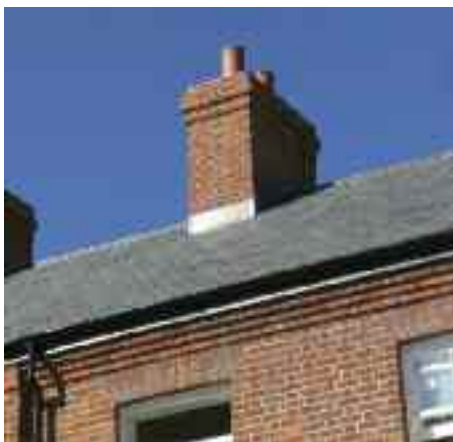
Chimney stack showing lead work. Also shown at lower level is brickwork corbel where airflow to the roof space is provided via a discreet corbel ventilator – see Ventilation section for details
