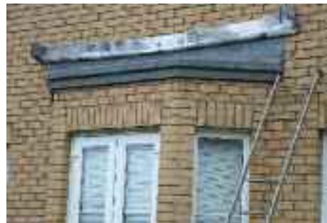
The extensive fascia height means there are a considerable number of masonry courses between the bay support lintel and the higher roof/tray intersection level. To prevent damp permeating between the two it is necessary to incorporate a vertical link whilst maintaining coursing and bond
