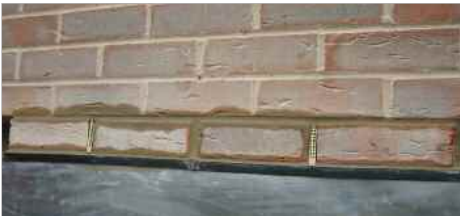
Type E Cavitrays with Type W Caviweeps
