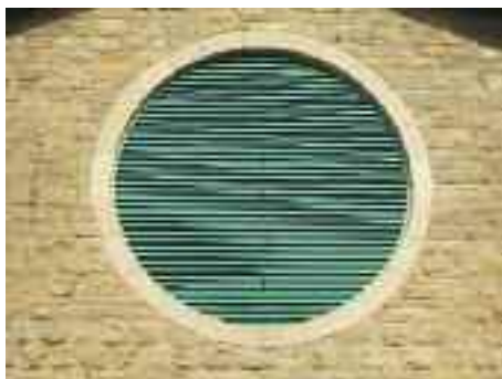
Circular ventilation opening
