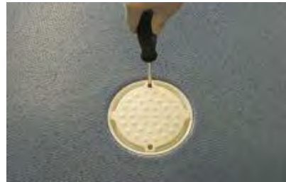
Remove 2 no. cap retaining screws. Do not remove clamp screws.
