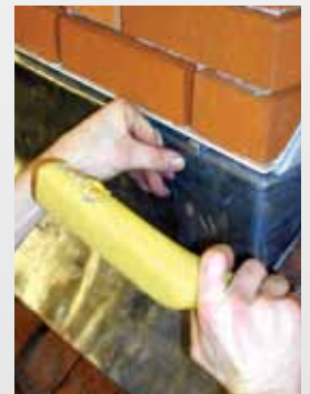
Step 6 The lead is then dressed securely into the flashing channel.
