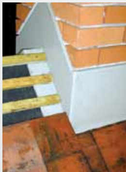
Step 4 Batten over the support plate as shown and tile the roof.
