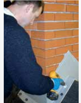
Step 3 Drill through support plates and screw to trusses using the fixings provided.
