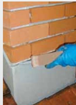
Step 5 Apply the supplied sealant to the channel before and after flashing.
