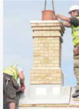
Step 2 Crane into position on the trusses using the lifting eyes and loops supplied.
