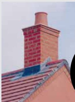
Step 7 Job done! The finished chimney is in place.
