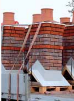
Step 1 Delivered to site ready for pointing (on the ground).
