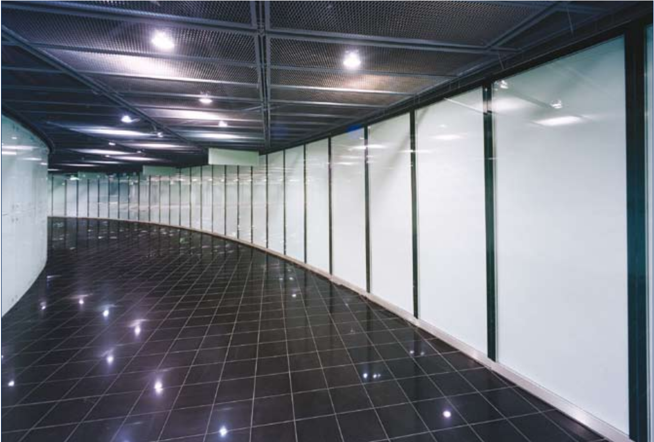
Passarelle, Sony Center, Berlin, Germany
