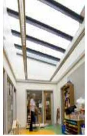
2 No. Multipart Flushglaze Rooflights with aluminium back to back angles The first rooflight - 1 No. 6822mm x 3000mm in 5 sections (wall abutted on 2 sides) had to be designed from scratch due to the split of the sections being uneven. The second rooflight - 1 No. 5995mm x 4000mm in 7 sections, also had to be designed due to non standard details being required.
