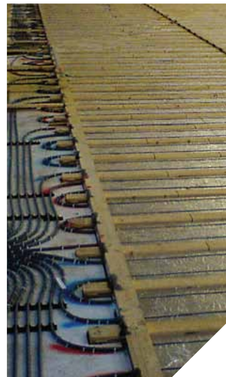
A unique sports floor underfloor heating solution is used in four West Kent colleges.
