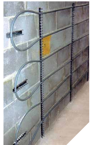
Special heating solution built into the walls at the RSPCA Kennels in Bath.
