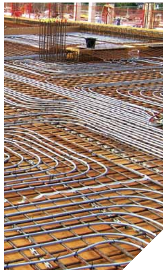
A unique and specific solution for in-situ cast slab as used in SGI Brighton.
