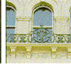
6. The finished elevation
