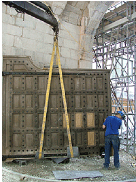
Re-hanging the gates to the Temple Bar after restoration
