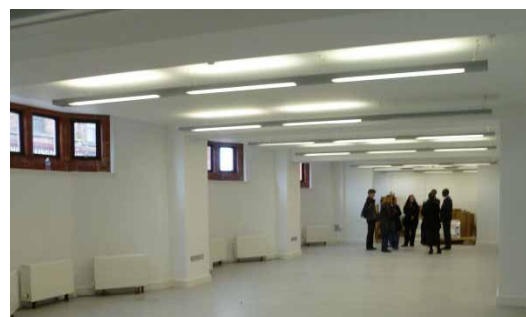
Newton 601 Flooring Membrane was used to seal the floors before finishes were applied
