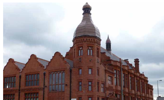
The Florrie, now fully waterproofed, will be officially reopened in July 2012
