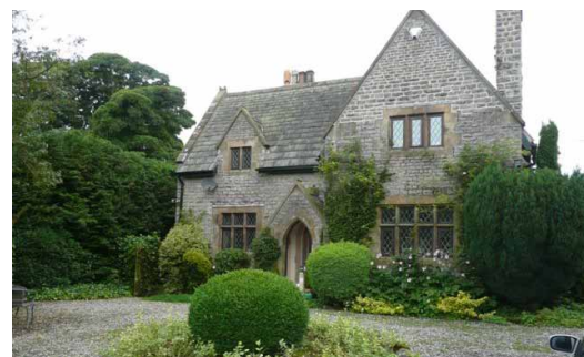
This listed property in Derbyshire is in a high Radon Gas area, so full gas remediation was required.
