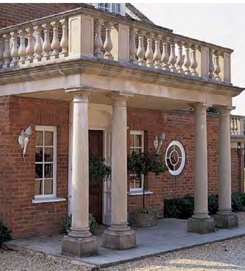
Portico D, M7 Columns and Balustrading.
