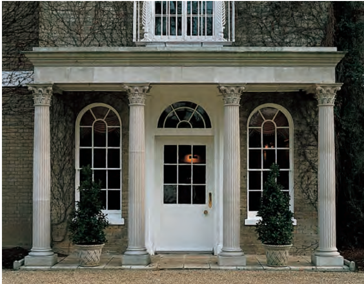
Portico E with additional Blocking Course and M2 Columns
