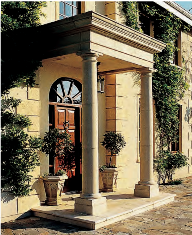
Portico A with M4 Columns, HN1 Steps and HN3 Risers
