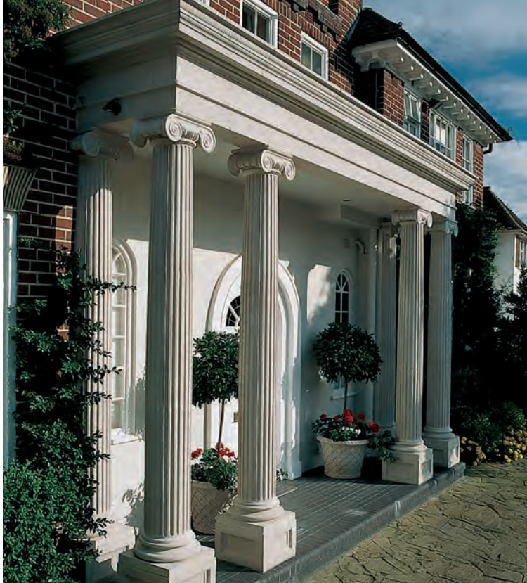
Portico A with M2 Columns.
