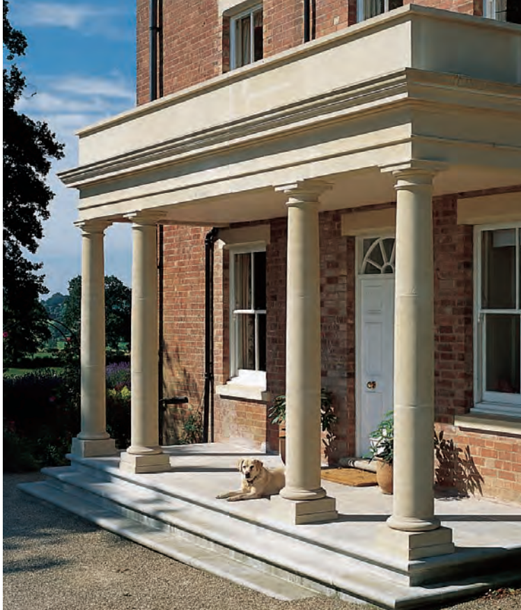
Portico A with M4 Columns, additional Plinth Block and Plain Parapet, HN1 Steps and HN3 Risers
