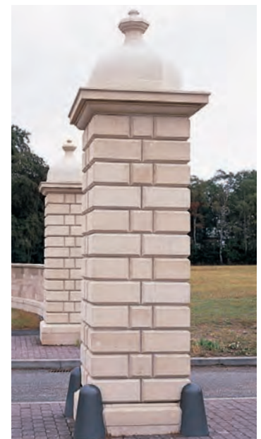
Custom gate pier.
