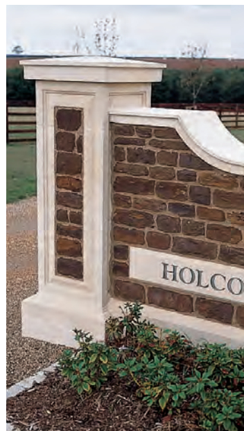
Custom gate pier.
