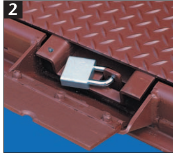
2 Recessed padlock hasp covered by a flush hinged lid
