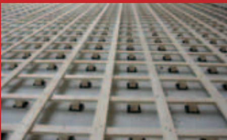
Installation of Harlequin WoodSpring at the Royal Ballet Studios, Covent Garden
