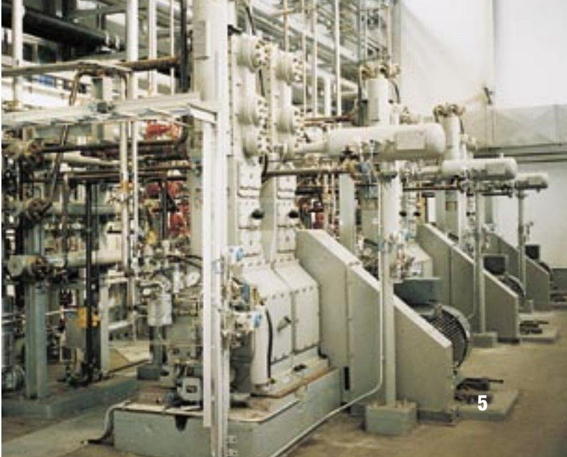
API 618 cylinder-lubricated or oil-free, either double or single compartment
