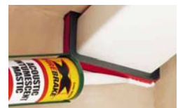
Intumescent mastic completes the perfect installation.
