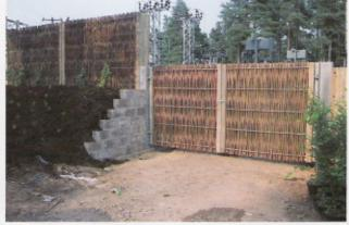
Sound attenuating gates incorporated, using the same high quality soundproofing material as the barrier.
