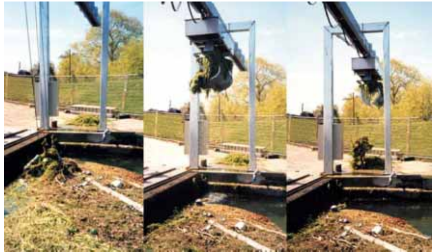
The Bosker Overhead Trashrake operating fully automatically under heavy debris conditions.
