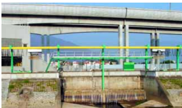
An installation in Hong Kong with two Bosker Overhead Trashrakes working over two intakes on a common track.
