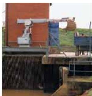
Bosker Bandit debris being dumped directly into containers for waste treatment or recycling.
