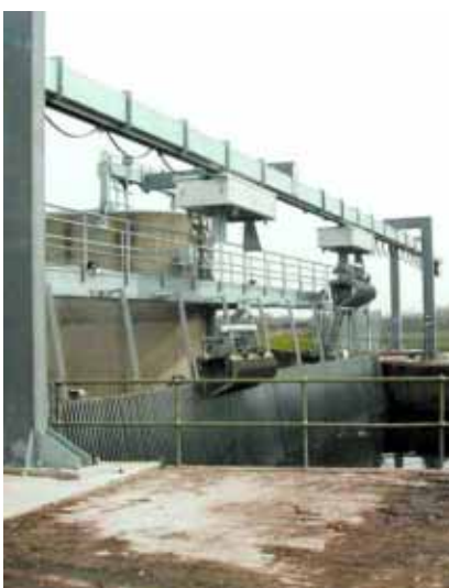
Eimco Water Technologies designed, manufactured and installed the above Bosker Overhead Trashrake with two machines on a common track each with a 3,000kg lifting capacity.
