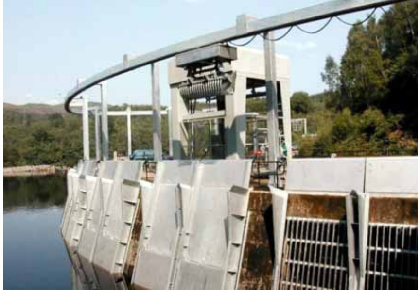
An Overhead Trashrake with curved track on a hydro-electric power station.
