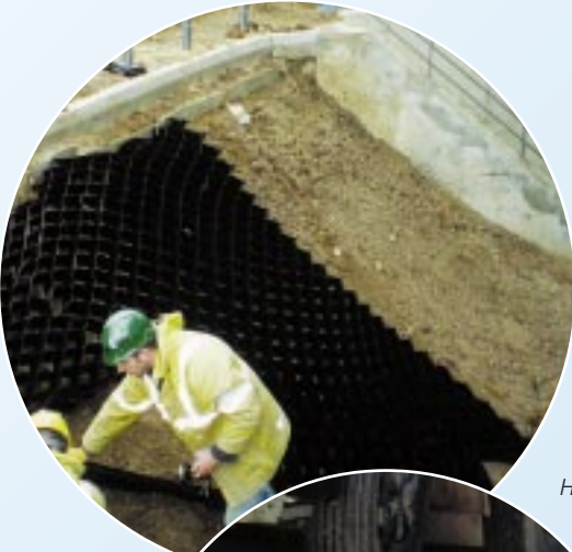
General embankment reinforcement Slough
