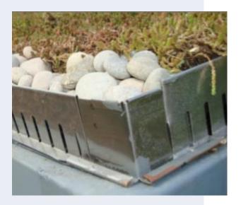
An aluminium edge restraint has a dual purpose, providing a restraint for the green roofing materials, but it can also be in-filled with pebbles, to provide an attractive feature to the installation.
