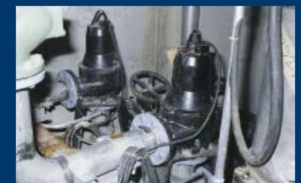
Vertically installed pumps, with stator housing conduit cooling.
