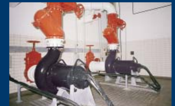
Horizontally installed pumps with cooling jacket
