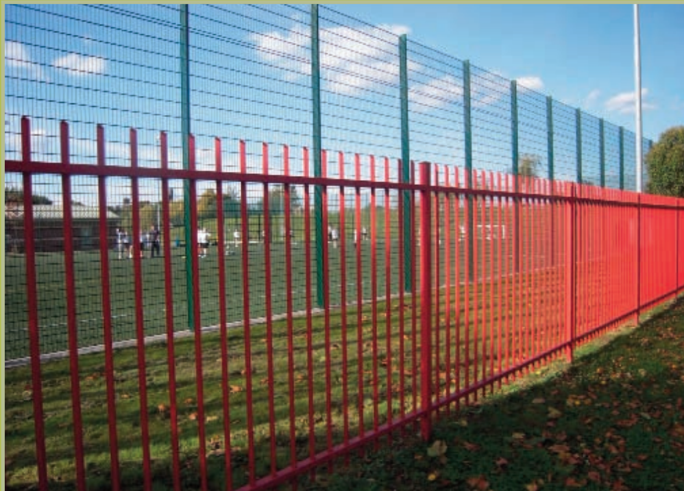
Sports mesh fencing, with railed fencing in the foreground
