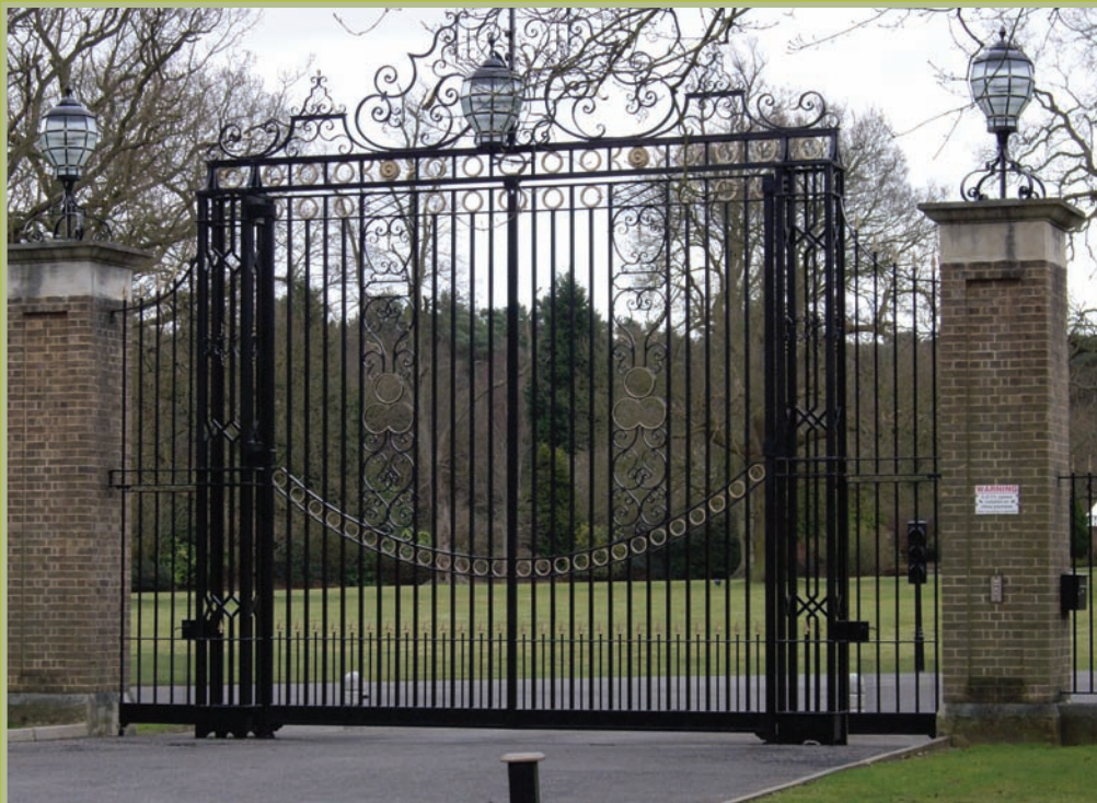
Bespoke 3 phase motor sliding gate, with a traffic light system
