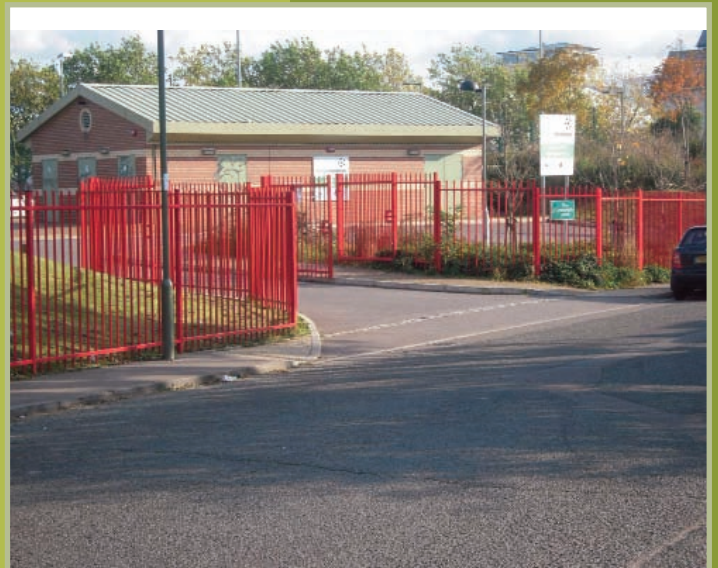
Railed fencing with gates
