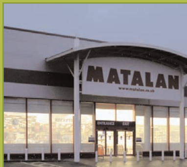
Perforated Steel Shutters
