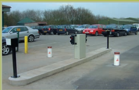
Twin automated bollard projects
