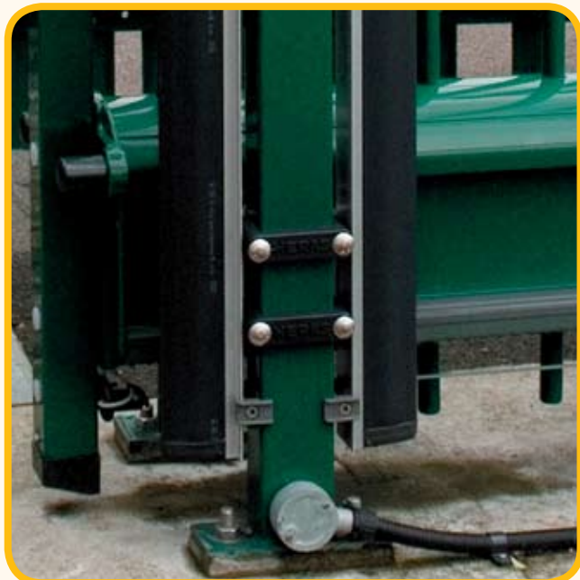
Bottom Running Wheels and Safety Edges
