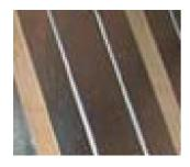
Grooved aluminium diffusion plates are fitted between the joists and the pipe laid in the grooves, insulation is fitted between the joists. The plates are fitted short to allow for the pipe to be looped
