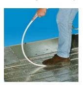
Pre-grooved insulation lined with aluminium to give effective heat distribution. The pipe is pressed into the grooves which clamp it in place. A baffle plate is fitted which incorporates the pipe bends.
