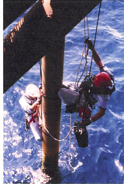
PEC inspection of a riser
