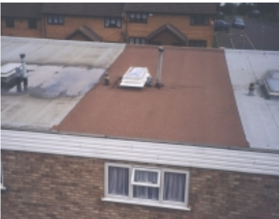
No water ponding
