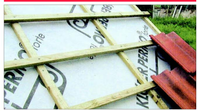
• THIS CERTIFICATE RELATES TO PERMO ROOF TILE UNDERLAYS, FOR USE IN TILED OR SLATED PITCHED ROOFS.
