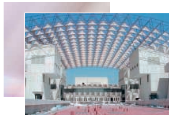
Ministry of Interior, South Surra (Kuwait) Calcium sulphate panels, 28,500 m 2
