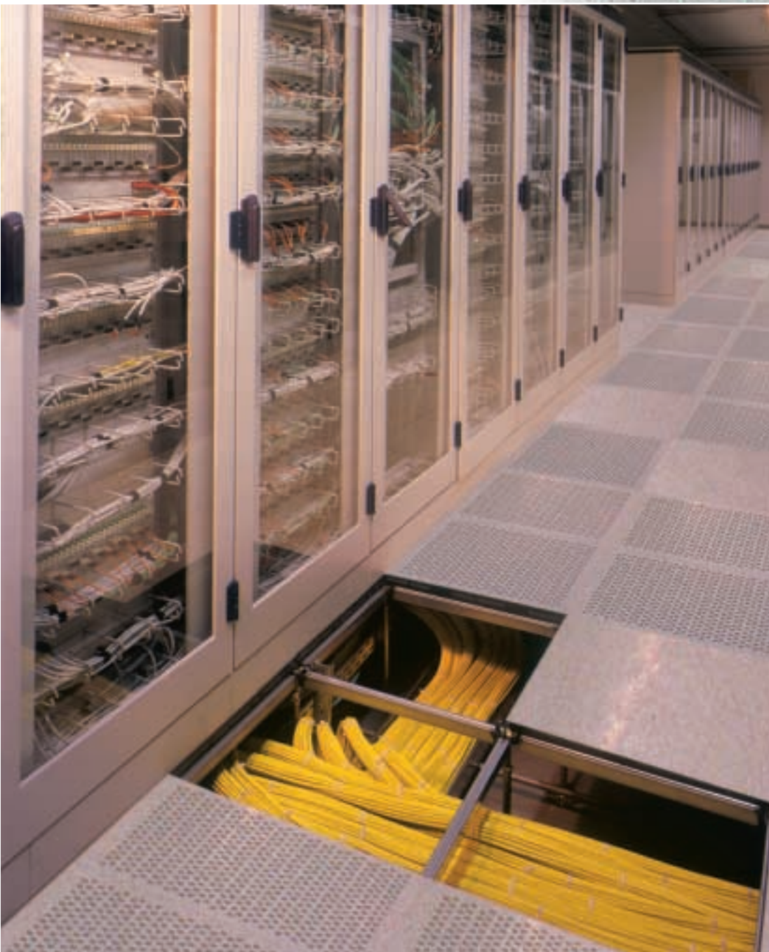
TechDataCenter, Munich (Germany)
