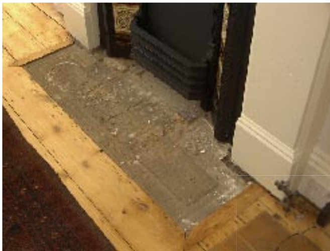
Fireplace to be restored
