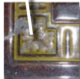
Relief design digitally reconstructed, 3D mould cut directly from computer and new tiles slip cast. Glazes matched to original.
