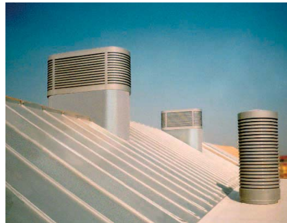
Top left: Indoor food market, Bridgetown, Barbados, where 10 No. 800dia Windcatchers were installed. The gentle offshore breeze provides the perfect driving force for these systems.
