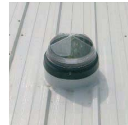
Alternative GRP upstand for British Steel type colour coated roofing sheet, bonded to surface
