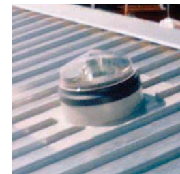
On-site welded upstand to Kalzip type roof with ABS collar
