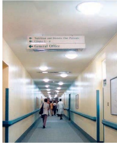
Top left: SunPipes serving the ground floor of The London Clinic, where the extension blocked off natural light to the ground floor windows.
