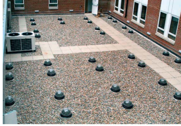
Centre right & lower right: Lewisham Police Station, London, where 50 No. 330mm diameter SunPipes were installed to the cells of this high security building. The SunPipe systems were fitted with vandal resistant top domes and security bars. Stainless steel ceiling trims were fitted with security screws.
