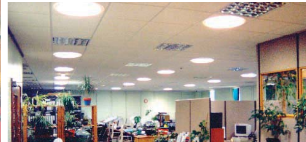
Top left: Library at Riverside College, Leicester, where existing rooflights were replaced with 14 No. 530mm SunPipes and 2 No. 600mm square Windcatchers, as shown in the photograph below. This eliminated the need for electric lighting during daytime and the need for air conditioning.
