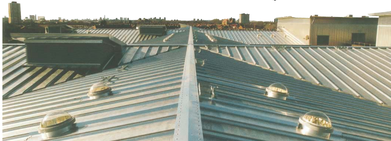
Lower right: 120 of our 530mm diameter SunPipes installed at Newham Hospital, London in 1998, to bring natural daylight down to corridors and Consulting Rooms.
