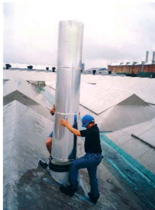
Top and Centre left: Sutton Arena, where 14 No. 750mm dia. SunPipes were used on the indoor athletics track.
