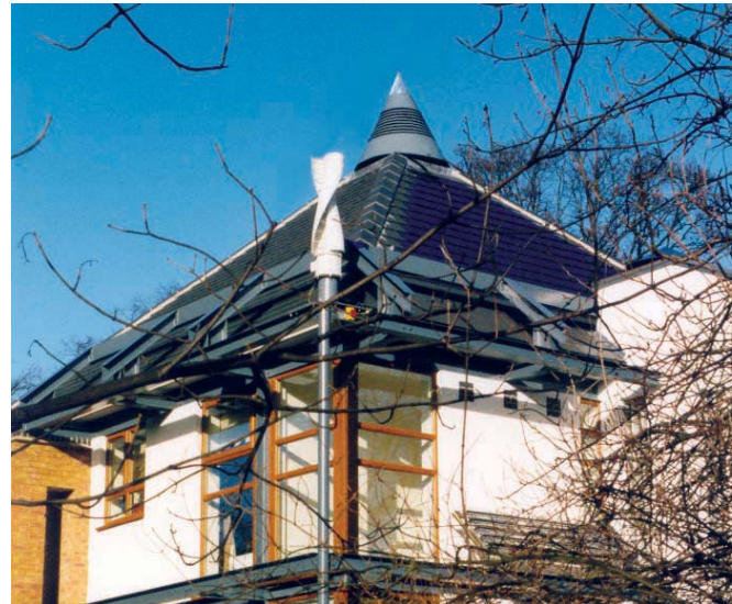
The 'famous' Eco House at Nottingham University which has had wide publicity in the Architectural press, featured a bespoke pinnacle SunCatcher system, with a polycarbonate cone. This highlights Monodraught's ability to produce any architectural feature. The pinnacle SunCatcher serves the first floor landing and staircase and a further SunPipe serves the ground floor cloakroom.
