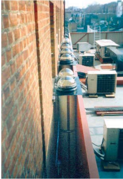
Top left: SunPipes serving the ground floor of The London Clinic, where the extension blocked off natural light to the ground floor windows.
