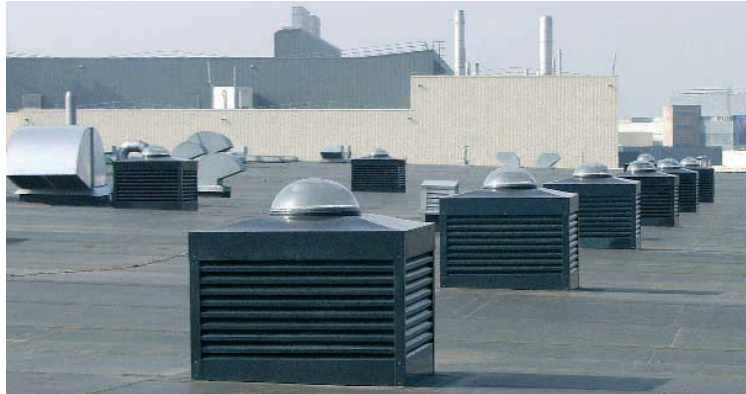
Top left: 26 of the 1200mm square SunCatcher systems installed at BMW Design & Facilities Offices at Cowley, Oxford.
