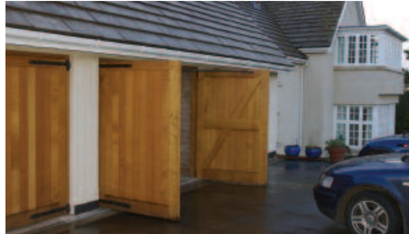
multiple garage doors on rendered garages
