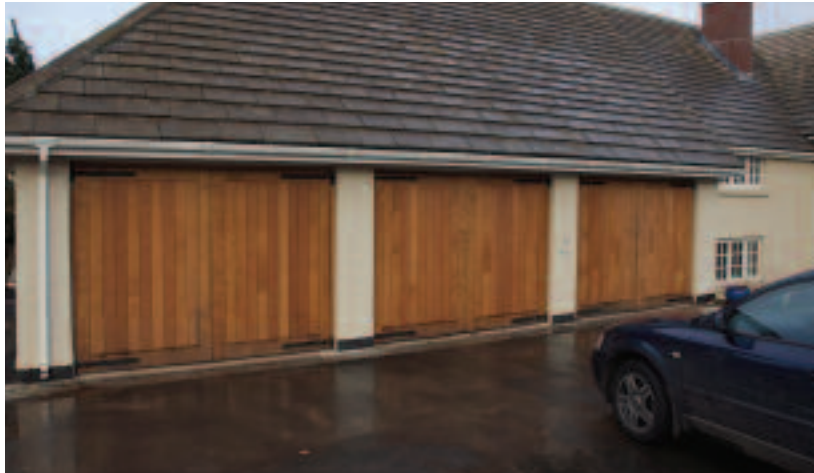
multiple garage doors on rendered garages
