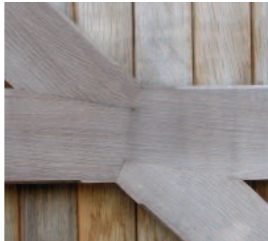
Kinnersley – brace detail (weathered)
