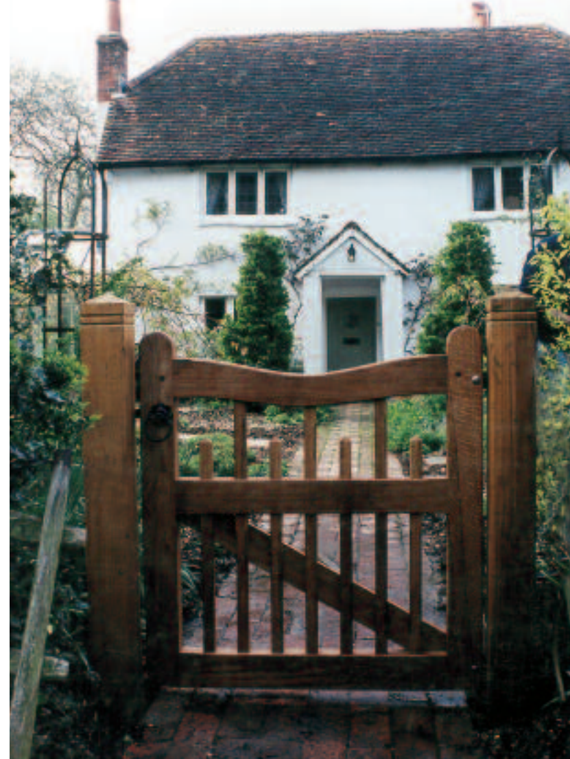
Brockhampton – falling curve
