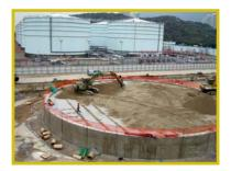
without damaging the seal across the body of the bund or at the numerous plinths and stanchion penetrations. Due to the simple installation procedures this user friendly system was easily installed by the contractors' own labour without the need for sub-contract specialist installers.
