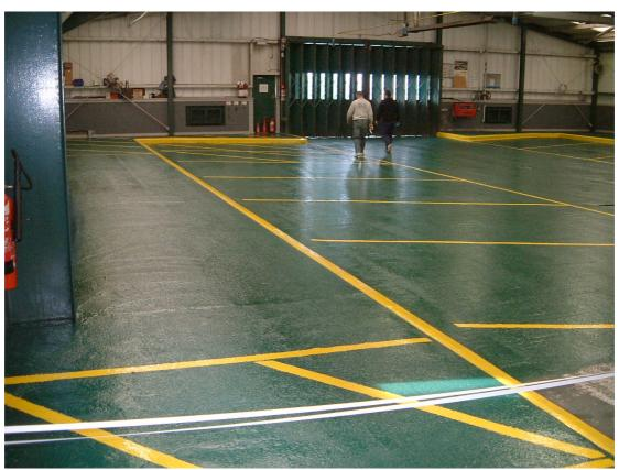
Just one hour later once the repairs had cured and hardened the first coat of RonaFloor HB100 Rapid was mixed with a drill and paddle and roller-applied. Ronacrete's anti-slip aggregate was cast into the first coat to provide the required degree of slip resistance for wet and or greasy floors. After only four hours the
