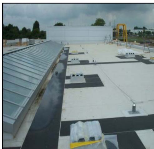
Demarcation of walkways
