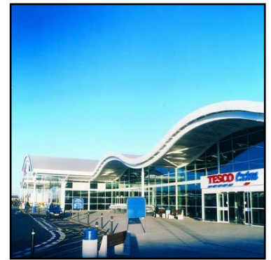
Tesco Plc – Kingston Park, Newcastle
