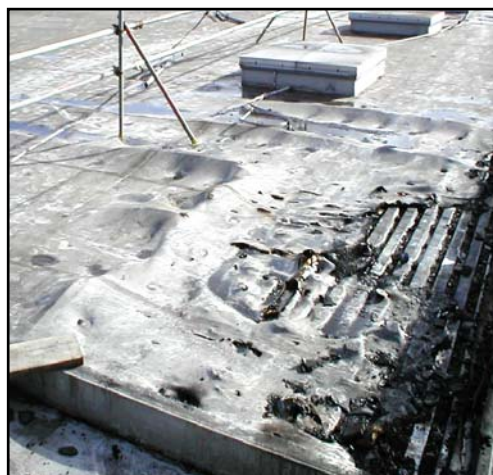
Fire damaged roof – only the Sika-Trocal membrane remains!
