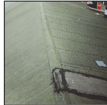
Deteriorated existing felt substrate
