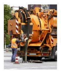
Traditionally, maintenance of an OWI would consist of a tanker with a 2 man gang extracting the whole volume of the OWI (in the case of even a medium sized OWI this could amount to 110,000 litres or 110 tonnes).
