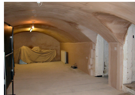
Completed Basement Waterproofing works awaiting decoration
