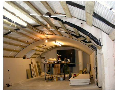
Basement Waterproofing Works in progress
