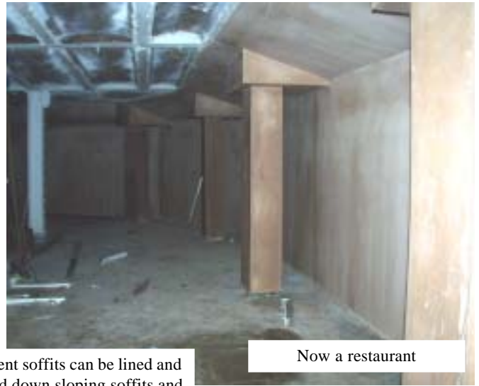
Cavity drainage technology was used to turn an unusable cellar into a comfortable and warm shop. Southport, 1990
