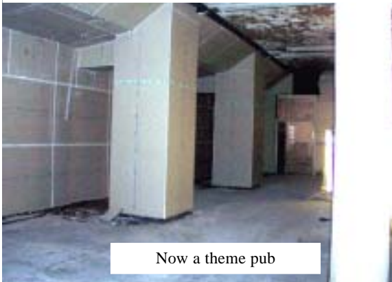
Showing how below pavement soffits can be lined and made dry, with water drained down sloping soffits and walls.
