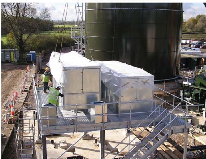
Outdoor installation of weatherproofed acoustic enclosure on centrifuge platform
