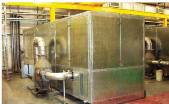
Indoor installation of acoustic enclosure around centrifuge
