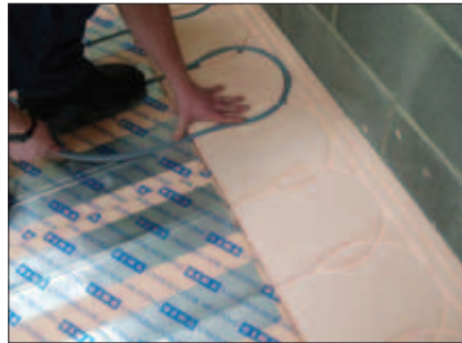
Floating Floor panel with integral heat diffuser plate
