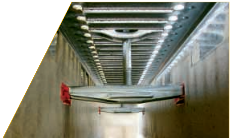
Fig. 19 PolyChannel SK Red Dot locking system
