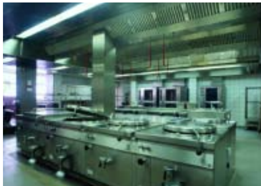
Typical Application. Bespoke Ventilated Ceiling.
