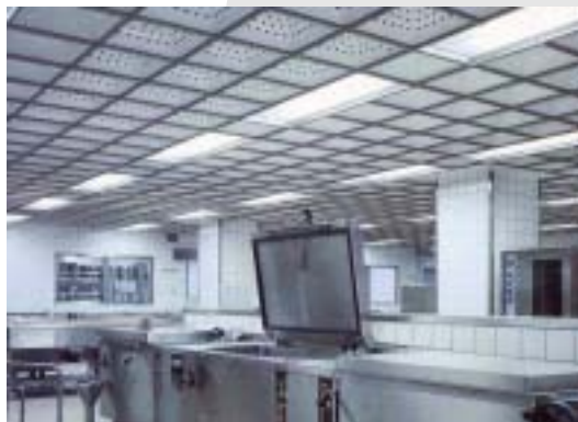
Typical Application. Cassette Ventilated Ceiling.
