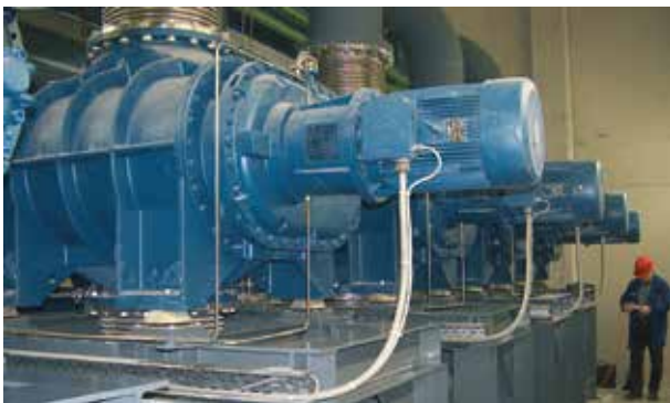
4-stage vacuum plant with 2 x 30,000 m 3 /h intake volume flow in steel degassing
