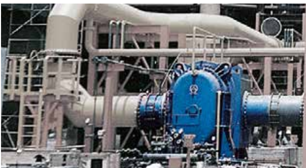
Plant for pneumatic conveying of bulk materials
