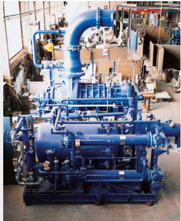
Soda Sanayii, Mersin (Turkey), compression of coke oven gas VRO 836 L, intake volume flow of 45.000 m 3 /h, compression of 0,85 to 3,5 bar (abs.), water-purged carbon labyrinth sealing
