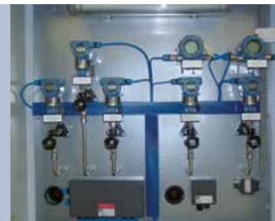
Intrinsically safe, specialized transmitter instrumentation – for use in hazardous zones
