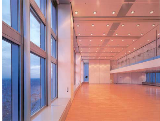
Plank Type Panels in the Open Plan Office Area
