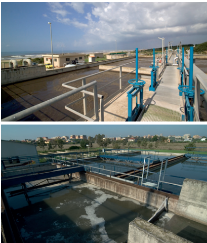
Acqualatina wastewater treatment plants
