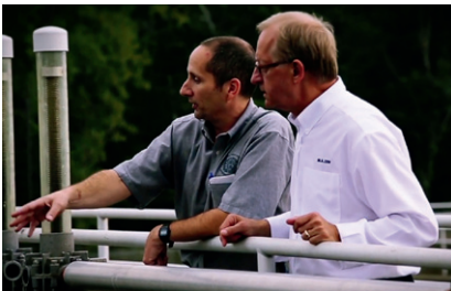
The wastewater treatment plant in Meriden
