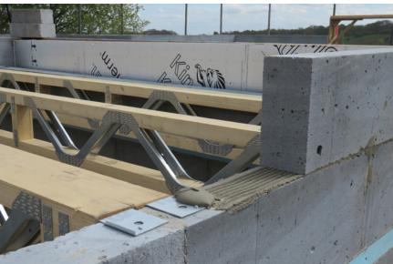
The wall U-value achieved was just 0.10 W/m²K with a construction of 150mm stone, residual cavity, 160mm Kingspan Kooltherm K8, 100mm Thin Jointed aircrete and drylining, as this provided good air tightness with the Thin-Joint system.
