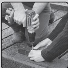
In fixing the profile to itself or other structures, it is advisable to condition for around 24 hours at ambient temperatures. Where possible, keep the profiles covered in their delivery packaging until use and try to fix at or near its maximum operating temperature.
